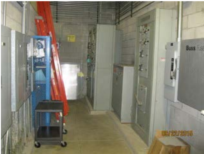
MDP/Transformer/Distribution Equipment
