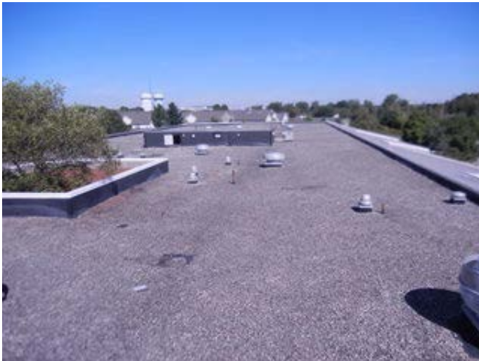
Ballasted EPDM Roofing
