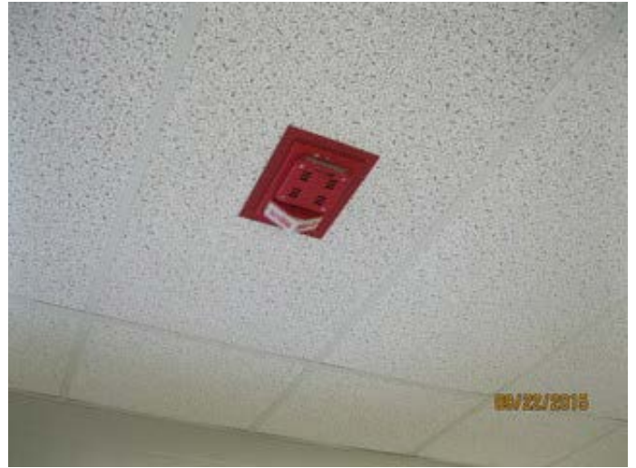
Ceiling Mounted Horn/Strobe
