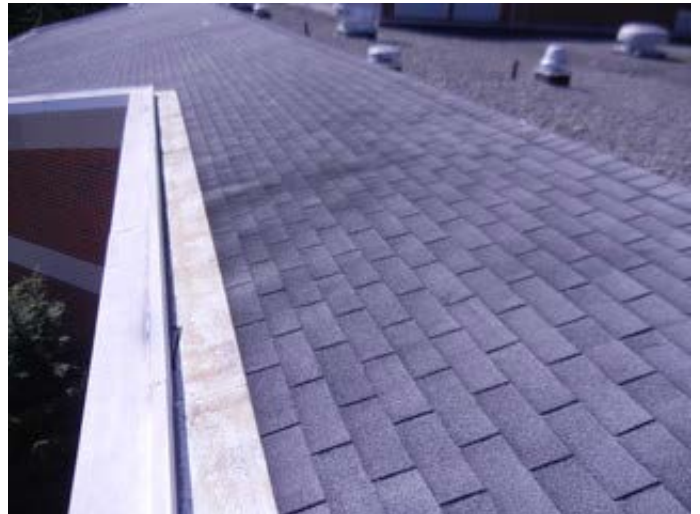
Fiberglass Shingle Roof
