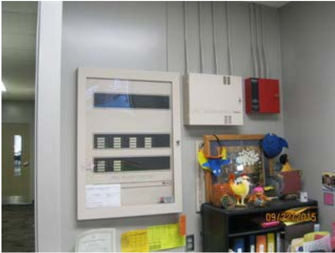
Fire Alarm Control Panel
