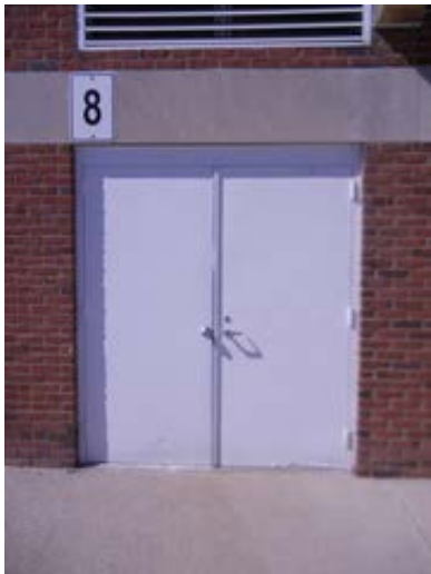
Typical Exterior Door with Inappropriate Hardware
