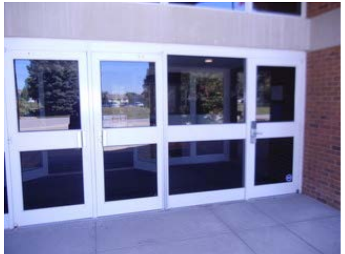
Curtain Wall System at Main Entry
