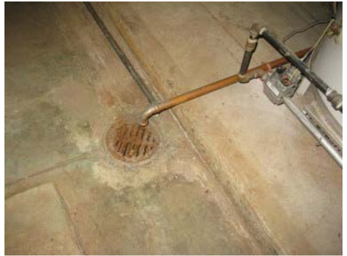
Exposed Waste in Boiler Room
