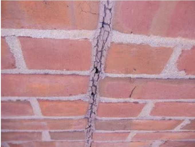
Typical Control Joint
